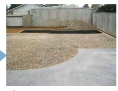
4. P-gravel compact into the honeycomb cells
