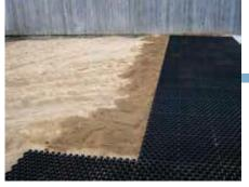
1. Prepare the base ground by removing overburden to form an even surface
